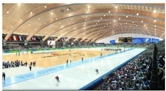
The one-of-a-kind five acre roof structure features hollow, triangular-shaped composite wood-steel arches, which span 310 feet and conceal mechanical ducts, electrical conduits and sprinkler pipes. Spanning between the arches are novel, prefabricated "wood wave" panels consisting of pine beetle kill 2 x 4's and plywood. The panels not only provide an economical structural solution but also a stunning aesthetic quality and enhanced acoustic performance.
