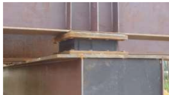
Fraser Heights Bridge – elastomeric isolation bearing.
