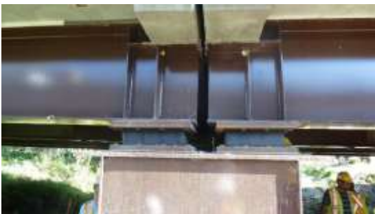
Fraser Heights Bridge – twin isolation bearings
