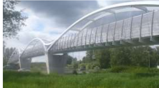
Tynehead Pedestrian Bridge – supported by twelve elastomeric isolation bearings
