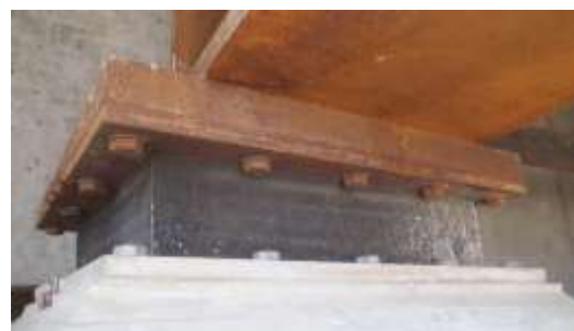
Elastomeric bearings at the Nelson Flyover abutments are 800 mm square and are key seismic load path components
