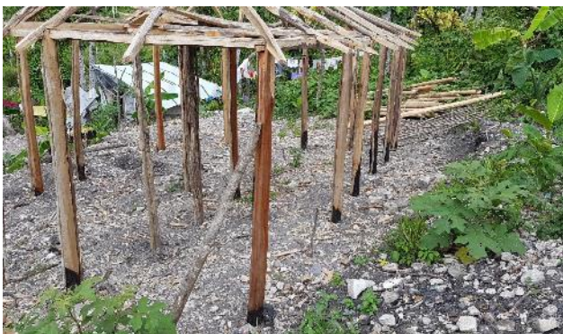
Figure 2. Post bottoms heated to pyrolysis so to reduce hygroscopicity for wood in contact with soil in traditional construction
