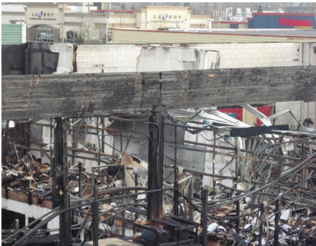
Figure 2. A char-damaged glulam beam surrounded by failed steel framing
