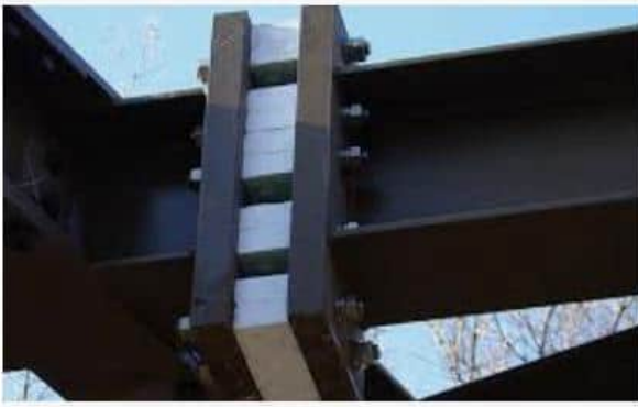
Thermal Breaks in Structural Steel.... uaa.alaska.edu
