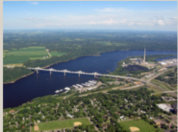
St Croix Bridge, Stillwater, Minnesota, USA, Length 1024 m
