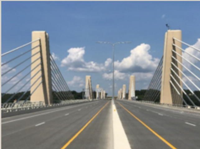
St Croix Bridge, View along the deck
